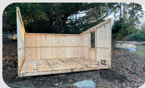
February: building the walls
