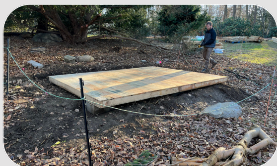
January: building the foundation
