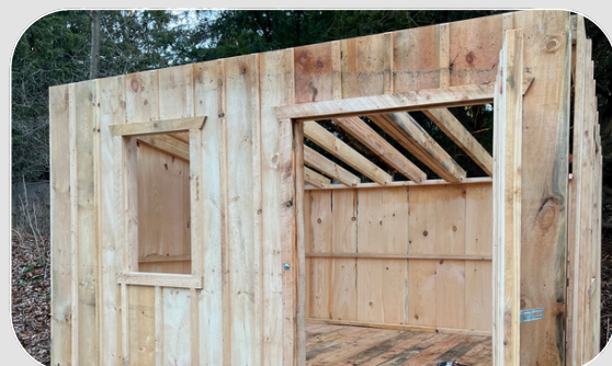
March: adding the roof
